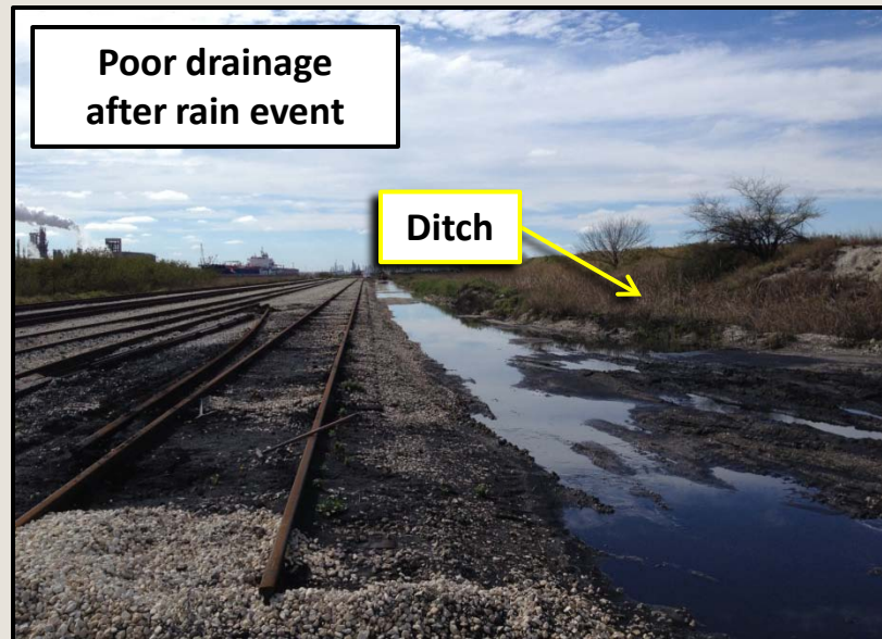
Soil build-up damming surface runoff
