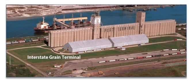
The Interstate Grain Corp. facility is capable of unloading 110-railcar shuttle trains. The elevator is served by the BNSF and Union Pacific railroads. Interstate's primary commodity export is wheat destined to Nigeria. Since Interstate is located beside the Union Pacific mainline, it is served direct by the railroad delivering the trains with no assistance from the Port Authority railroad (CCTR). The Port Authority collects half wharfage tariff on cargo at the Interstate dock.
